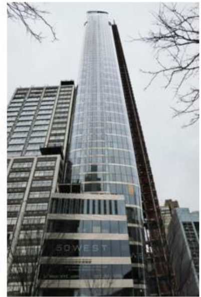
50 West is expected to be ready for partial occupancy at the end of the year. Photo: Carl Glassman/Tribeca Trib
