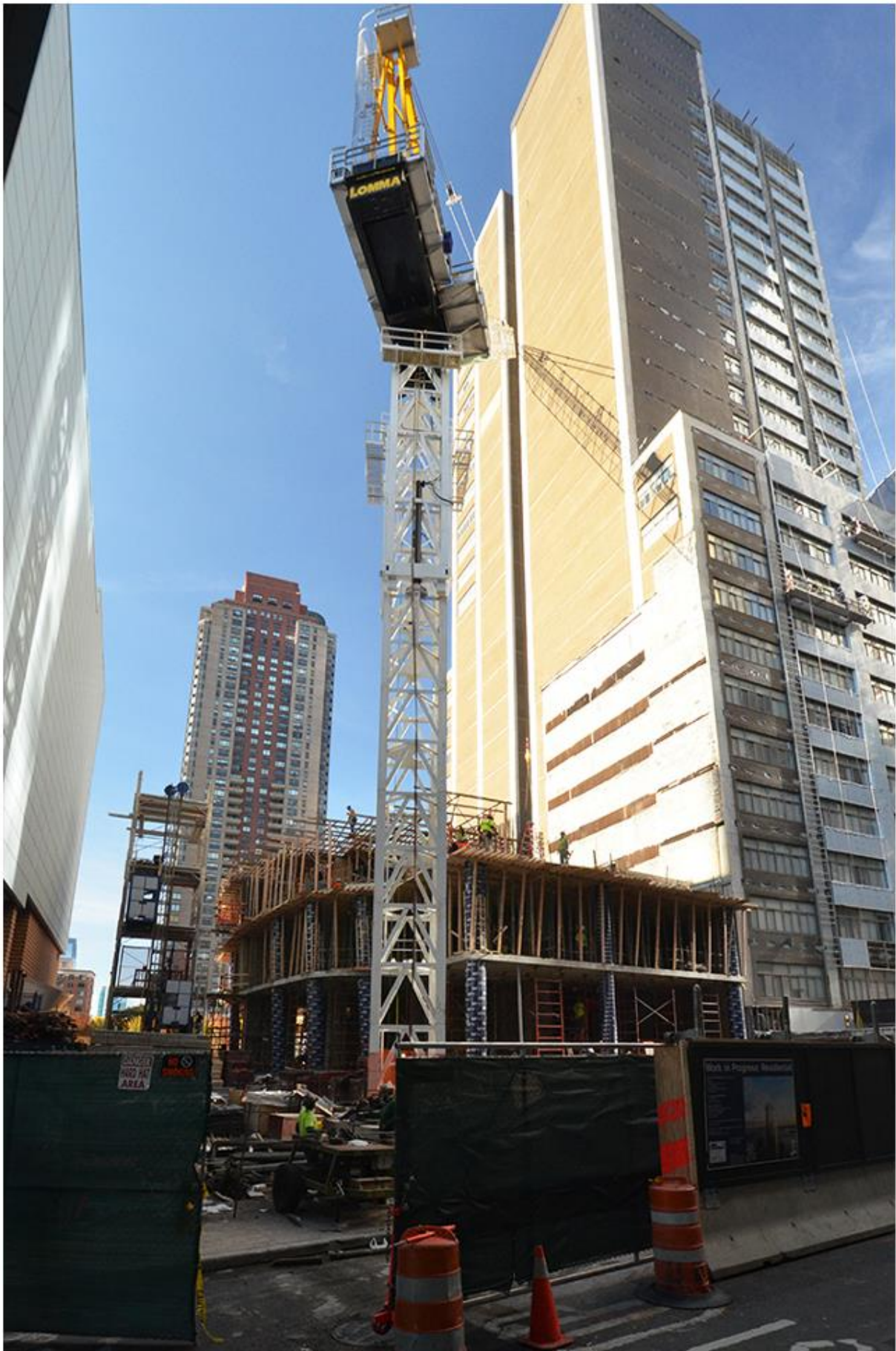
50 West Street, photo by Tectonic — 90 Washington at right
